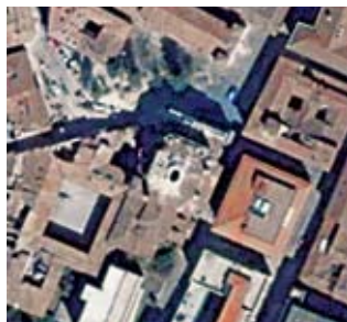
AFTER: Bell tower collapsed Collected April 8, 2009
